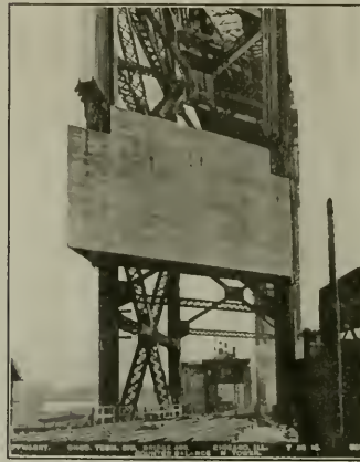
NORTH TOWER OF BRIDGE, SHOWING COUNTER BALANCE
